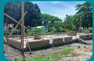
▲ Construction of a community-built triple-classroom project in Port Resolution, Tanna Island
