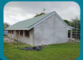
▲ Construction of a double-classroom for Amaro Primary School on Lelepa Island, Shefa Province
